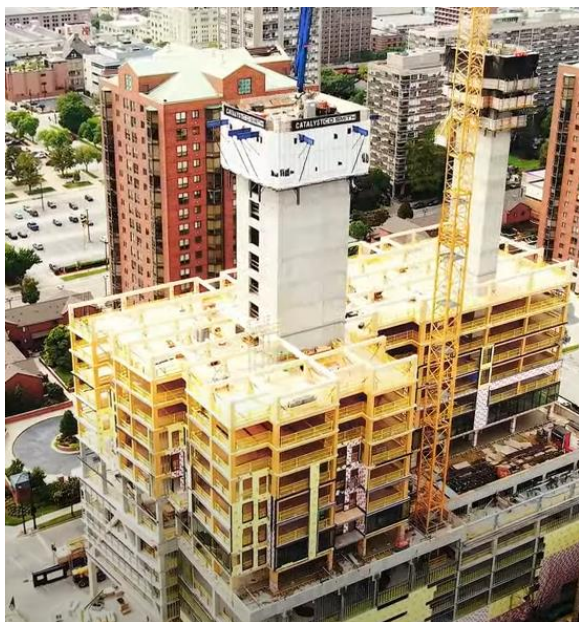
Non-timber op. 1: Concrete shear walls
