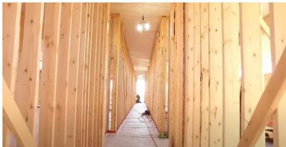
Timber op. 1: Light-frame shear walls
