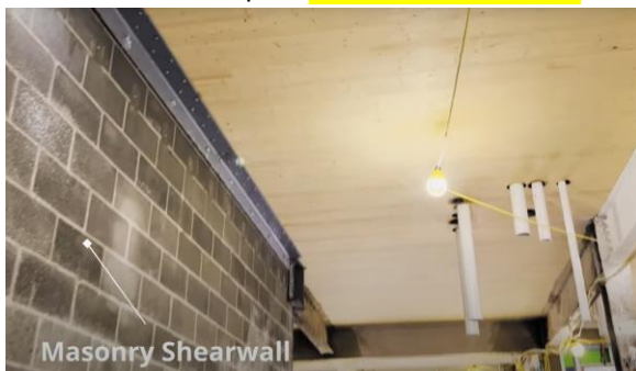
Non-timber op 3: Masonry shearwalls
