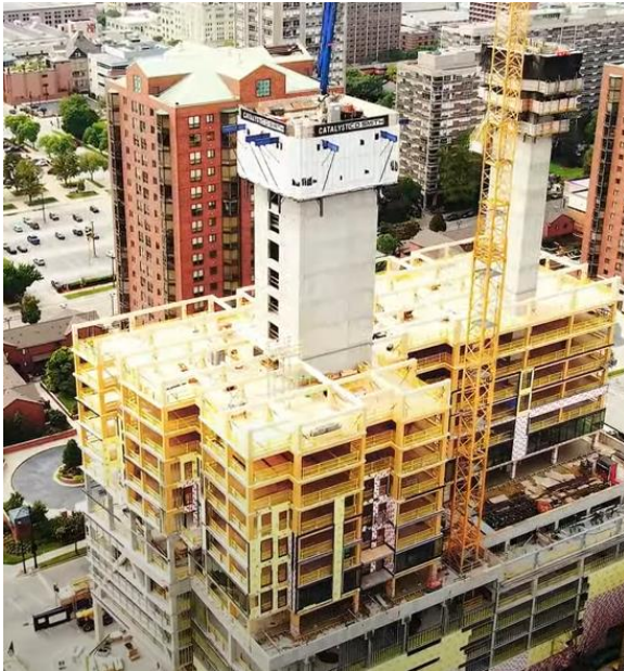
Non-timber op. 1: Concrete shear walls
