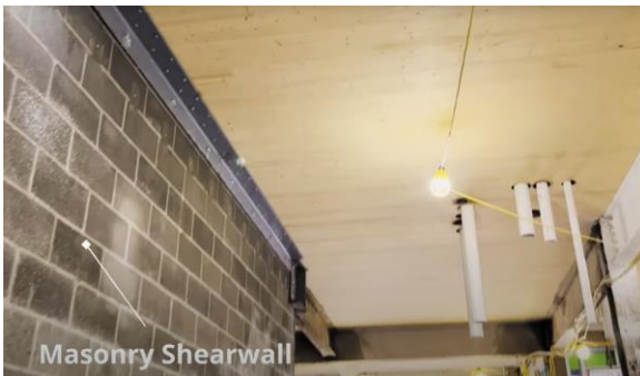
Non-timber op 3: Mansorary shearwalls
