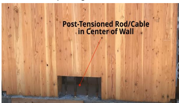
Timber op 3: Mass timber rocking shearwalls
