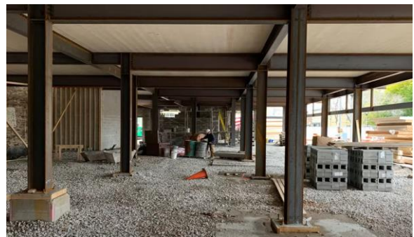
Non-timber op. 2: Steel braced/moment frames
