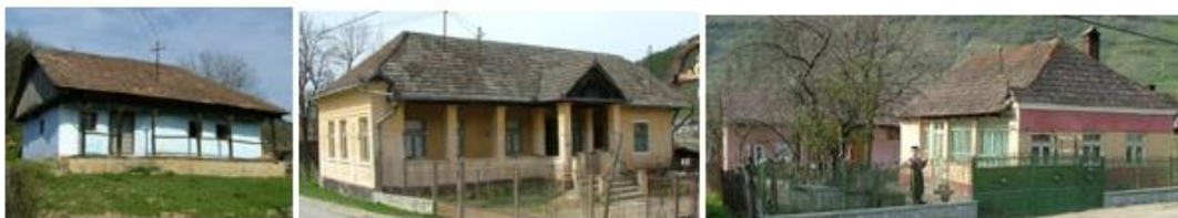
Figure 21 The first image is a traditional wood architecture. The terrace of the house with a southern orientation is an open space. The terrace covering protects the entrance door and windows from overheating of the sun
