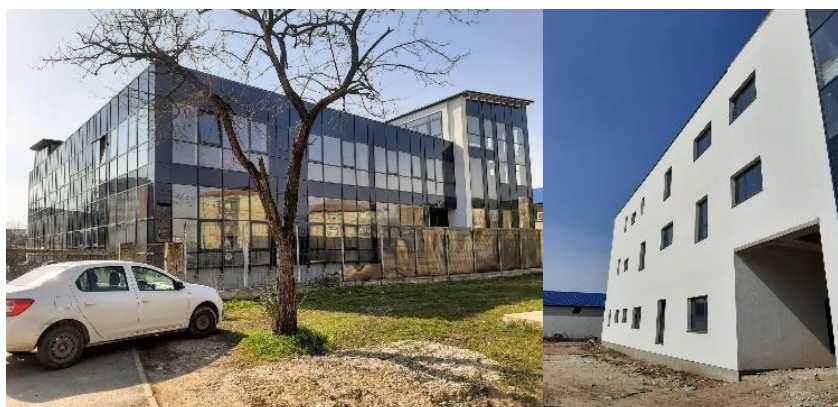
Figure 12 Project Concept Ditoiu Nina-Cristina-photos 27.05.2021, Ditoiu Nina-Cristina, The Curtain facade is to be shaded with vertical sun visors, Corian color White, initially with color inserts
