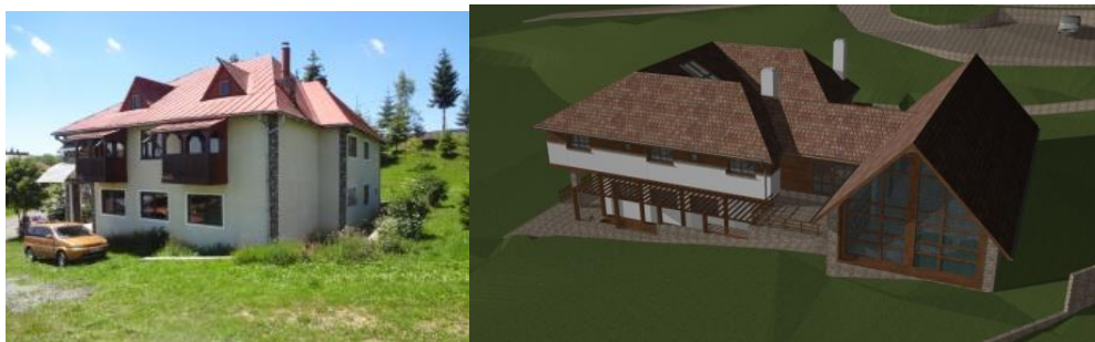
Figure 17 Project Dițoiu Nina-Cristina, Inspiration for rehabilitation and extension of house with square courtyard, project 21 : The first image is the original guesthouse building, an architecture built in the 1990s as a rehabilitation of a traditional smaller house. The second image is a rendering with the proposed building for the extension and redevelopment of the farm stay with space for the indoor pool
